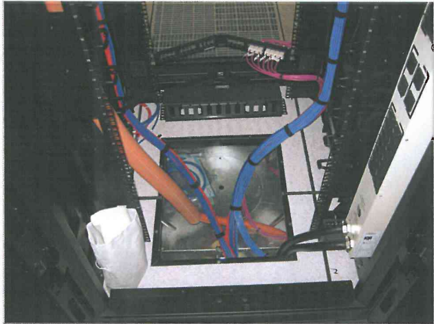
Tier E/A™ allows for generous cable cutouts without the need for burdensome gaskets
